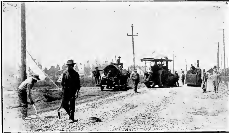
Work on Sacramento and Folsom Road. Ransome-Crummey Co.
